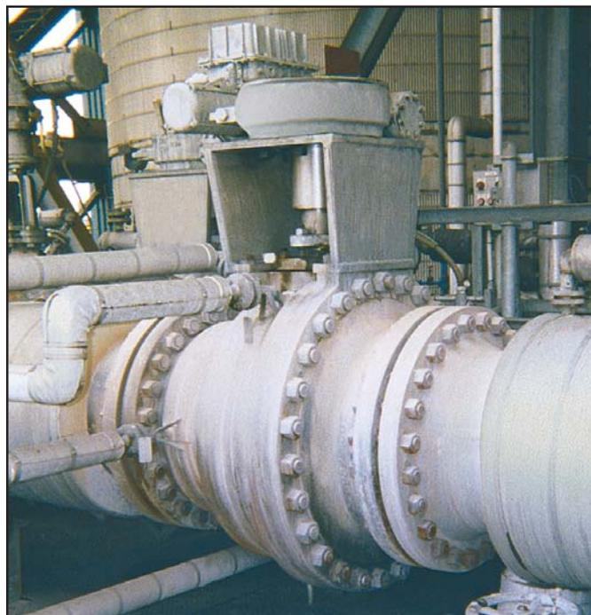
*These 24" full bore overhead vapor valves have been in uninterrupted service for over 6 years. In an effort to maximize liquid yield Delayed Cokers worldwide are opting for larger overhead lines. In fact some of the newer DCU's have already installed our 30" valves for overhead and blowdown service.*
