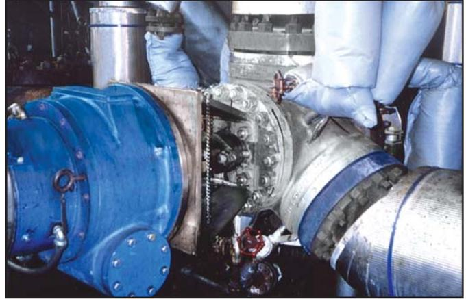
*The adjacent photograph shows a 12" switch valve installed with the stem in the horizontal position. The valve is installed in a delayed coker unit, where the valves were interlocked through a DCS for safer operation. Our logic control panel allows the valve to be operated both locally or remotely.*
