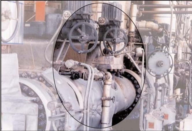
*This patented Velan Ring Valve was installed to replace an existing butterfly valve. The end user required the use of this valve only when shorter cycle times required quicker drum "backwarming". The end user could not justify the high pressure drop across the butterfly valve with his efforts to increase liquid yield. They required a valve with good throttling characteristics, but which provided no obstruction in the full open position. The Ring Valve fully met these requirements.*
